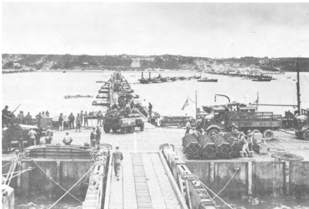
COMPLETED PIER OF THE MULBERRY in operation. Loaded vehicles coming ashore, above, and leaving Lobnitz pierhead, below.
