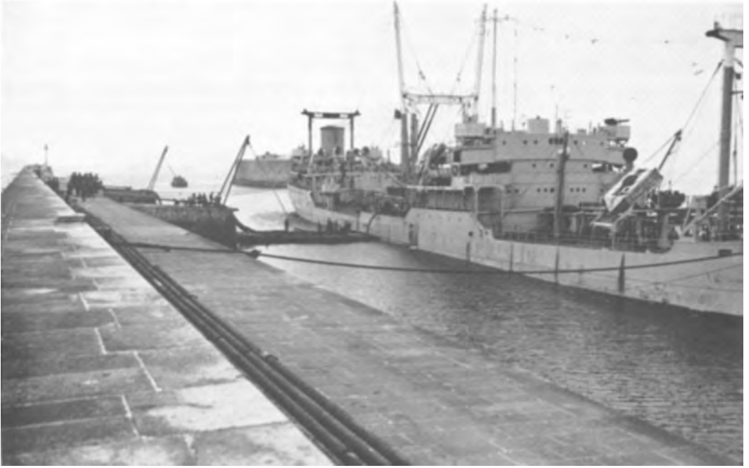
THE FIRST POL TANKER alongside the Digue de Querqueville , Cherbourg, 25 July 1944.
