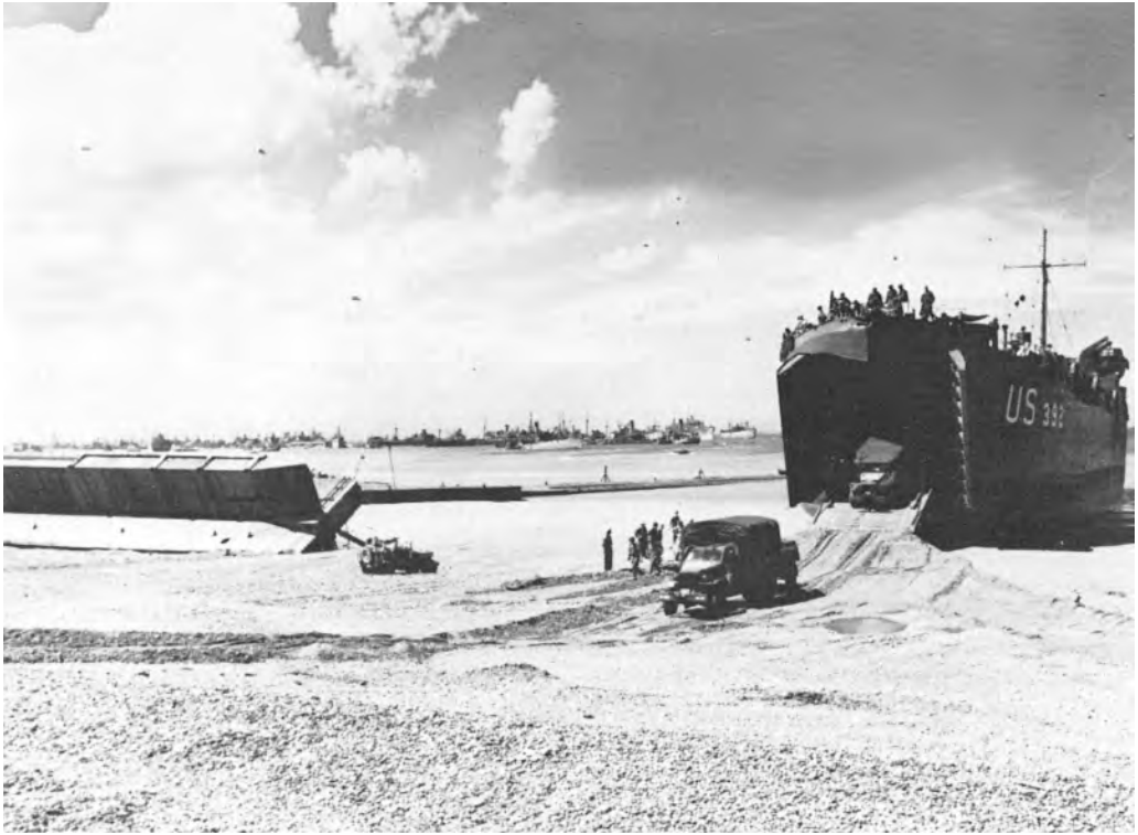
DRIED-OUT LST discharging its cargo at OMAHA Beach. Portion of a BOMBARDON washed ashore during storm may be seen at left.
