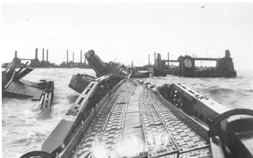
STORM-TWISTED PIERS. Lobnitz pierheads are visible in the background.
