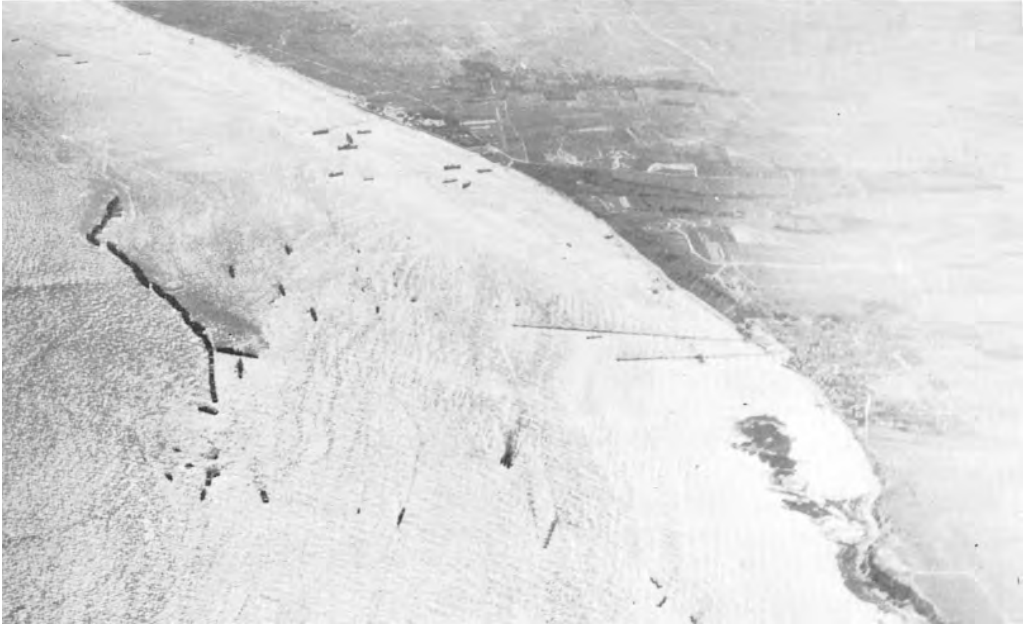
PARTIALLY COMPLETED MULBERRY off OMAHA Beach . Portion of breakwater, above; piers and pierheads, below.
