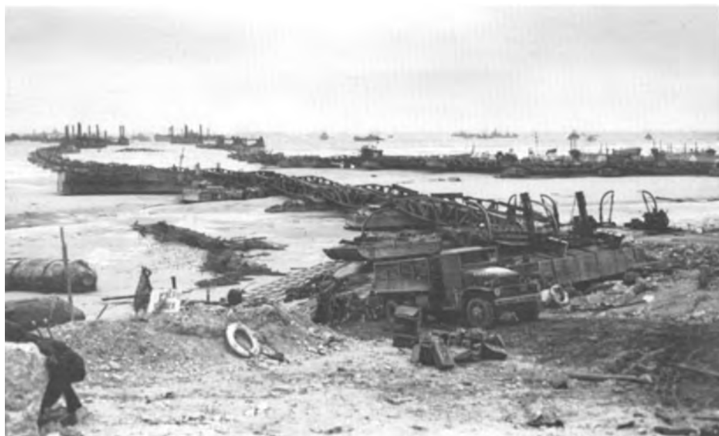
STORM-TWISTED PIERS. Lobnitz pierheads are visible in the background.
