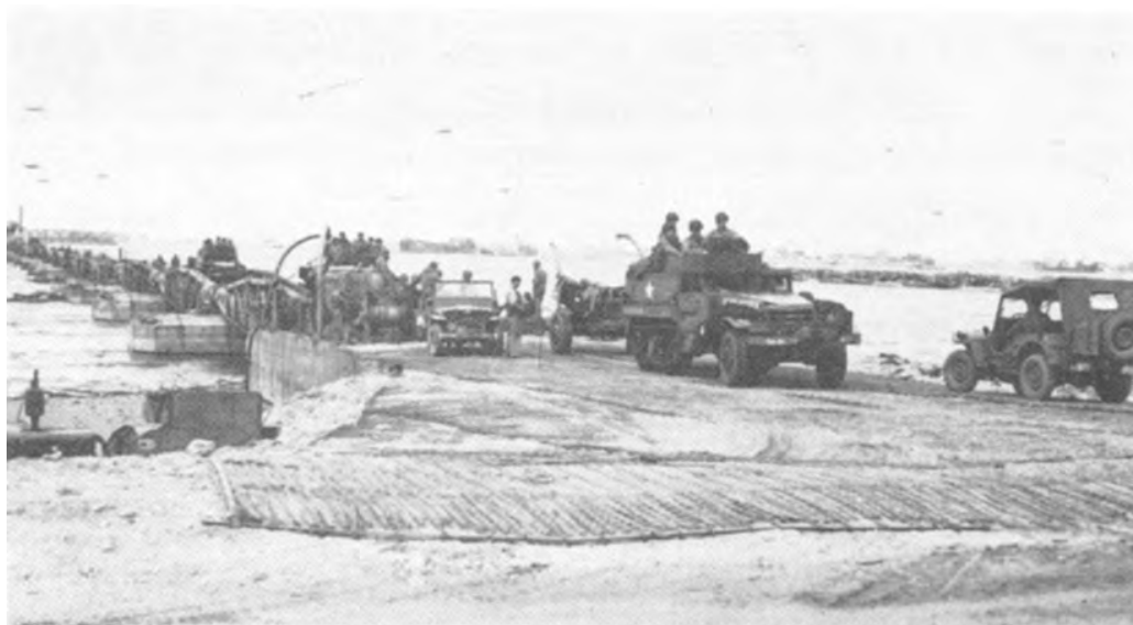
COMPLETED PIER OF THE MULBERRY in operation. Loaded vehicles coming ashore, above, and leaving Lobnitz pierhead, below.
